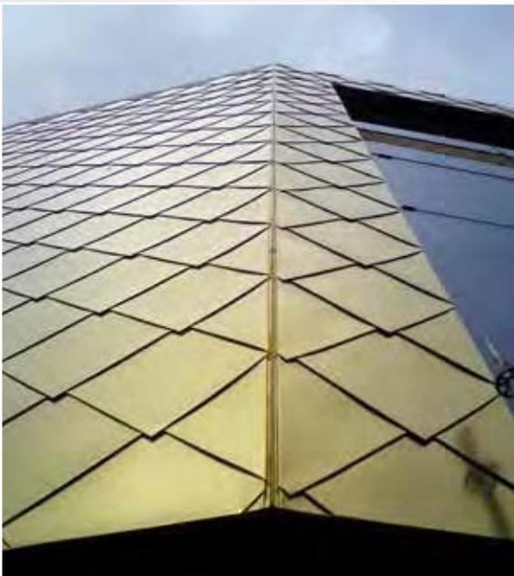
All horizontal changes of direction for both elevations and the roof cones (with one exception) were expressed with a raised corner.
