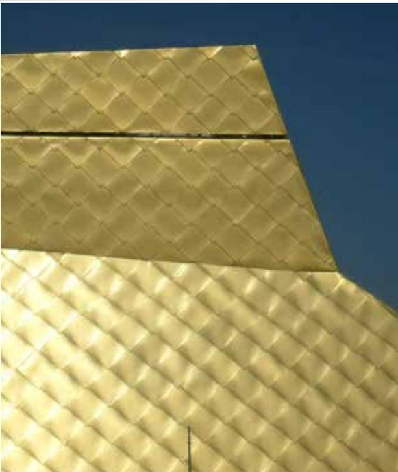
From the outset, the roof intended to have a horizontal break that gave a datum against the various pitches and roofs. It also demarks the upper and lower baffles. It is an expressed 100 mm gap, across which the shingle pattern appears to be continuous.
