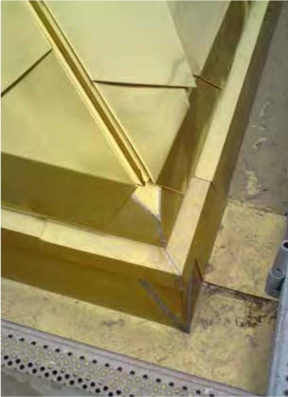
The roof hip is subtly different to the elevation hip – to prevent water ingress it essentially forms a pair of secret gutters that run either side of the central 'pro-w'.
