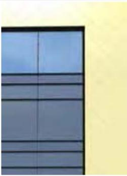
The copper alloy cladding was to appear 'thin', as a drape or fabric, with a reveal thickness at the glazing of only 25 mm.
