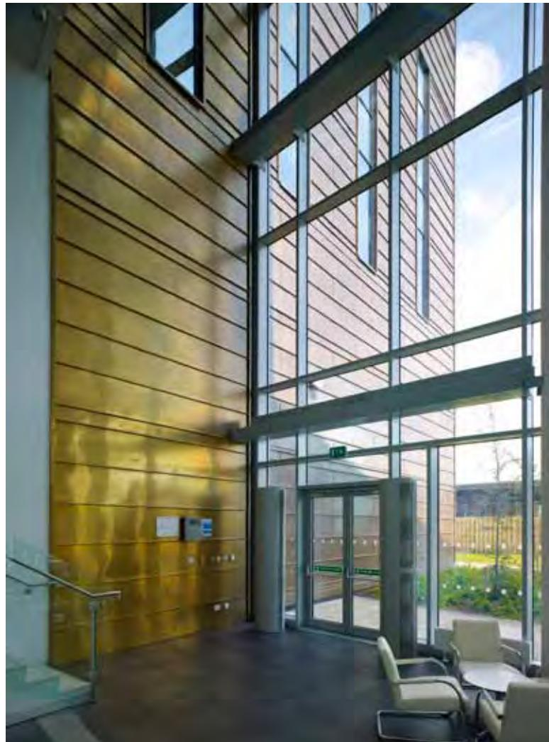
*"By providing varying textures of materials and cladding modules the volumes have taken on an expressive independence. This theme was further developed by using pre-patinated green copper to clad the curved walls of the auditorium. The boundary between internal and external spaces has been blurred by the continuation of the copper and brass cladding inside the building."*
