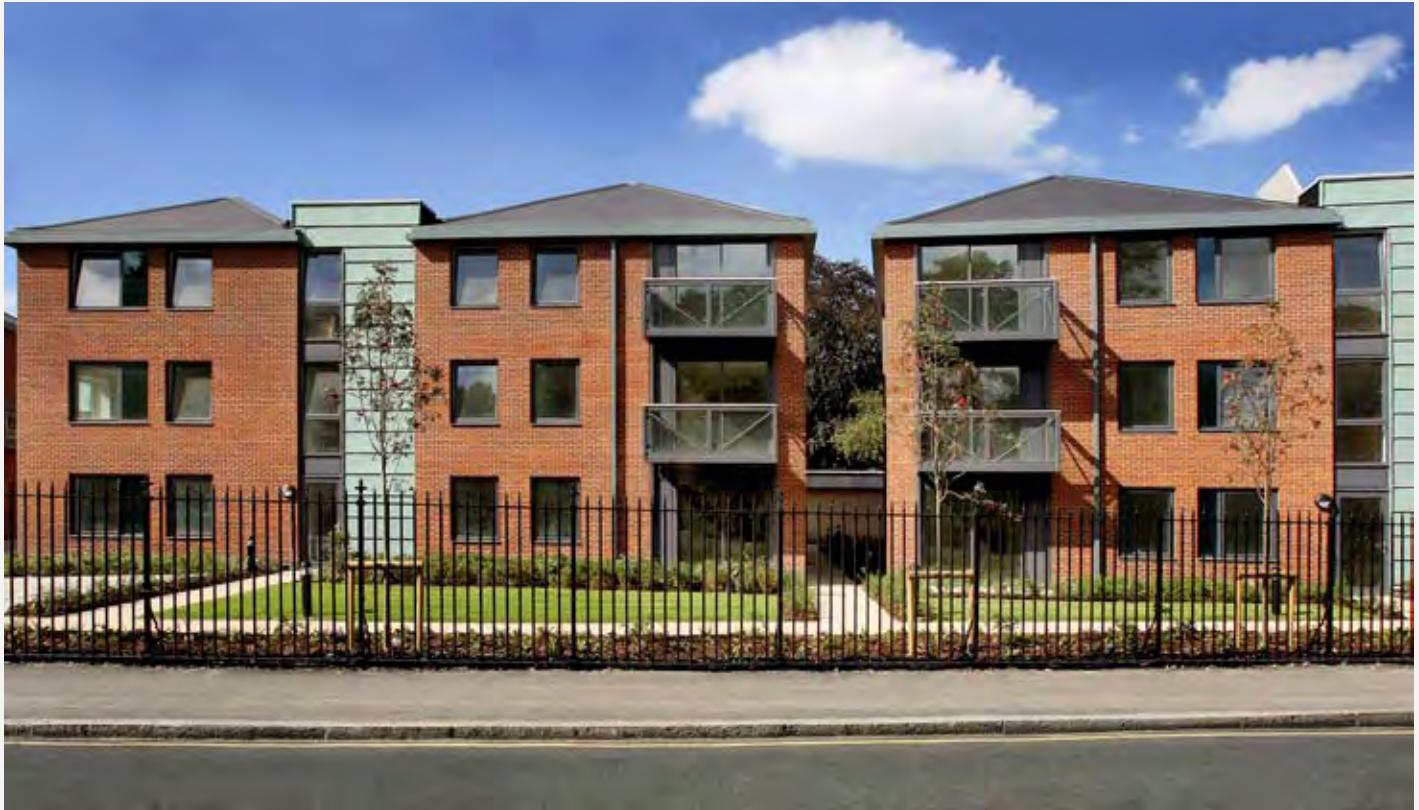
Vertical stacks of pre-patinated copper rhythmically punctuate the block elevations.
