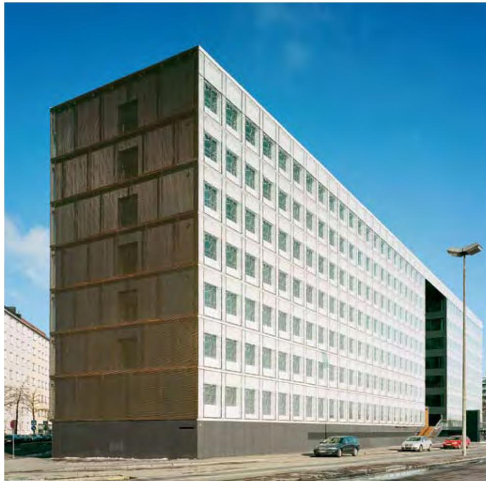
The copper façade, view from west. The transparency of the copper net varies to some degree according to lighting conditions.
