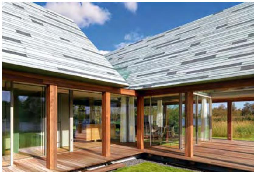
one another – define the building. Their surfaces have been devised using pre-patinated copper of three different intensities of green speckled against a dark oxidized background. These varied colours are used in a composition of long, narrow copper strips with different widths to give a rich, natural texture. Beneath one roof volume is the living room while the other sits over the bedrooms and an extra bathroom.
